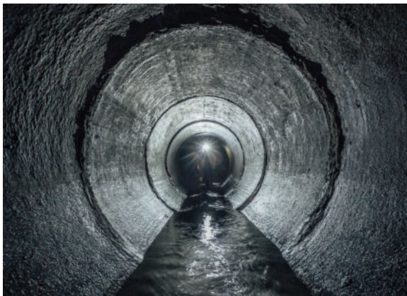
Interior view of a sewer pipe (Source: Mulderphoto|stock.adobe.com)
