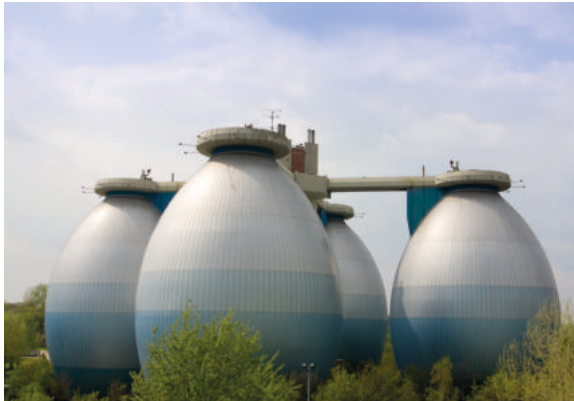
Wastewater treatment plant with digestion towers (Source: Arnd Drifte|stock.adobe.com)
