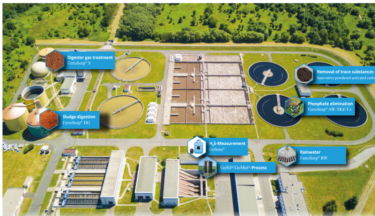
Aerial view of a wastewater treatment plant, individualized with possible applications of products from HeGo Biotec GmbH (Source: peteri|stock.adobe.com)
