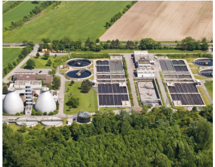
Wastewater treatment plant (Source: Thomas Leiss | stock.adobe.com)
